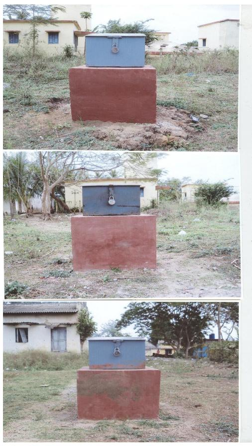
Protection Box (Plate thickness GI sheet -. Annexure-Q 3.00 mm) 65 CM 65 CM 53 CM 45 CM 55 cm 55 CM 25 mm ¢ holes **Bottom Side** 10CM 55CM 35CM X 5 CM 10CM 65 CM 5 mm Heavy duty Hinges Heavy duty pad lock SIDE VIEW 53 CM 45 CM
