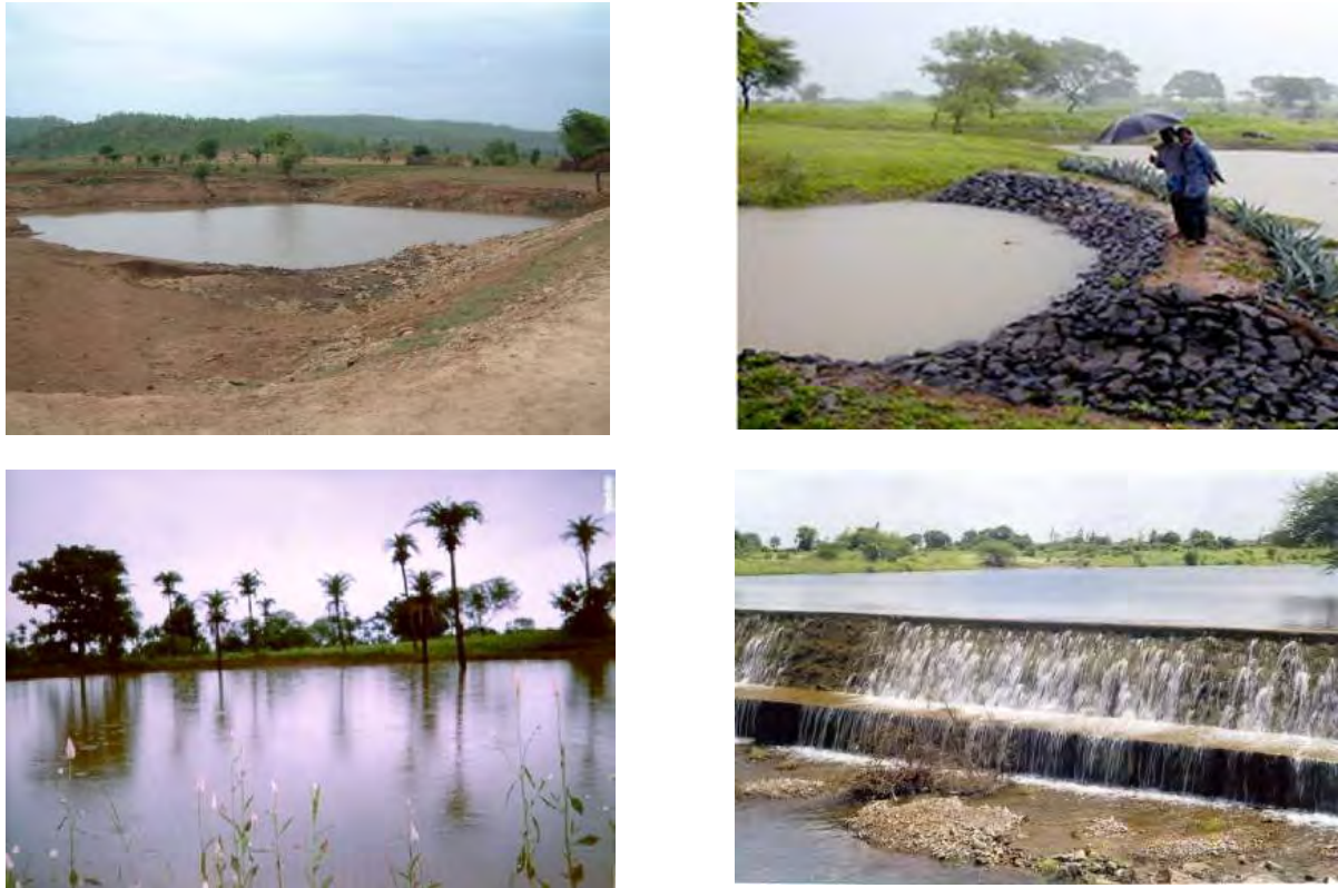
Figure 1. Runoff harvesting structures constructed in community watersheds in India.
