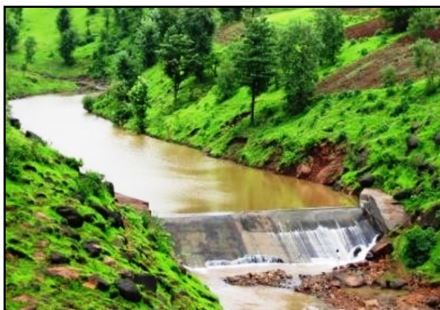
Figure 10.2 c : Illustrative Check Weir in Operation
