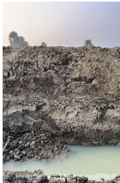
Clay formation up to 4 m at excavation near Rafiganj.
