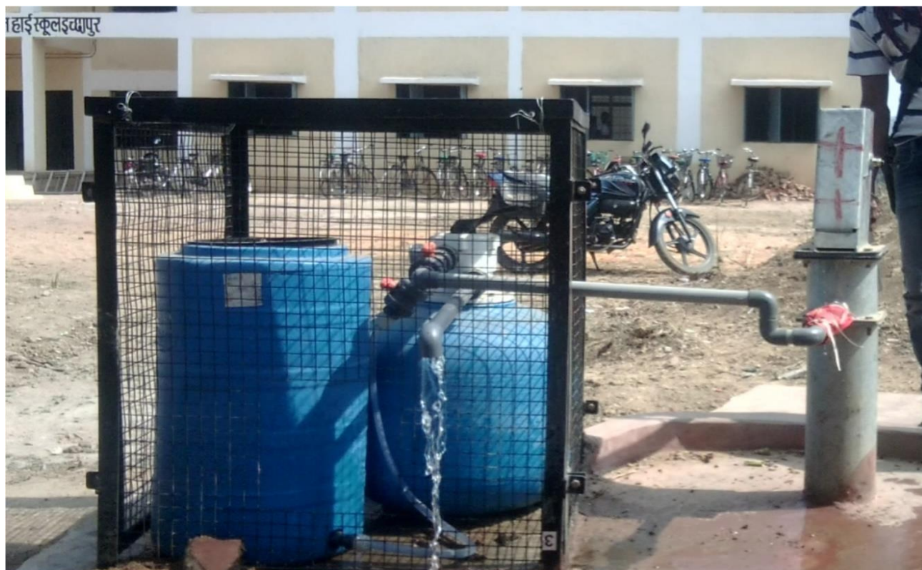
Figure 60: De-Fluoridation treatment plant attached to Hand pumps tube wells, specification evaluated by NEERI (National environmental engineering research institute) Nagpur.
