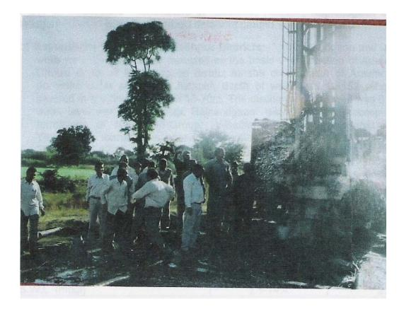
A high discharge Zone (16 lps) struck at depth of 263 meters in a dry area (Deccan traps ) at Athner, Betul (M.P.)
