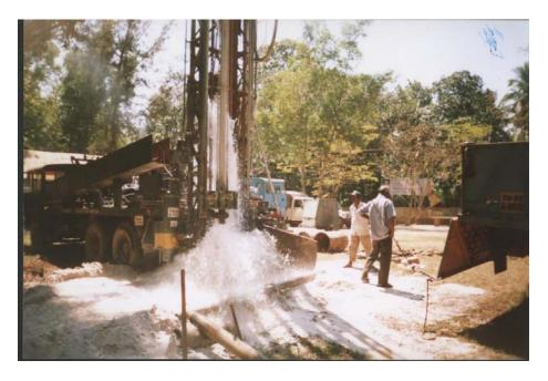
Drilling of Exploratory well at Malayadi, Trivandrum District with a discharge of 7.0 lps. Rock type: Garnetiferous gneiss
