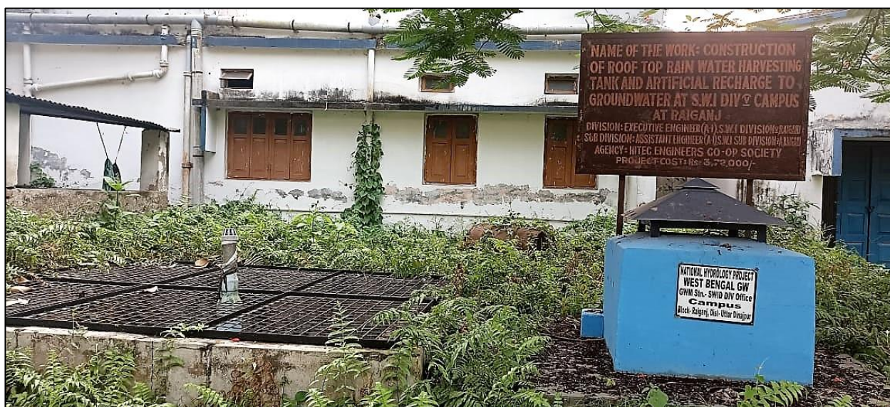
Roof top rainwater harvesting and artificial recharge project in SWID Division-V Campus, Karnojora, Raiganj block. SWID piezometer with AWLR system is seen in the foreground.
