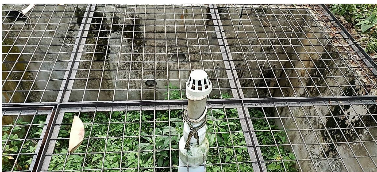
Close up view of recharge well and rainwater harvesting tank in SWID Division-V Campus, Karnojora, Raiganj block.
