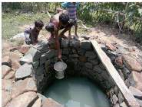
Photo 13: A stone walled dug well near Childa, Patna block never dries in a year.
