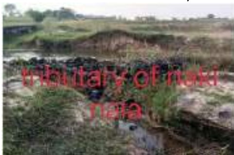
Photo 15: The gabbion structure for water conservatiuon over Naki nala in Patna block
