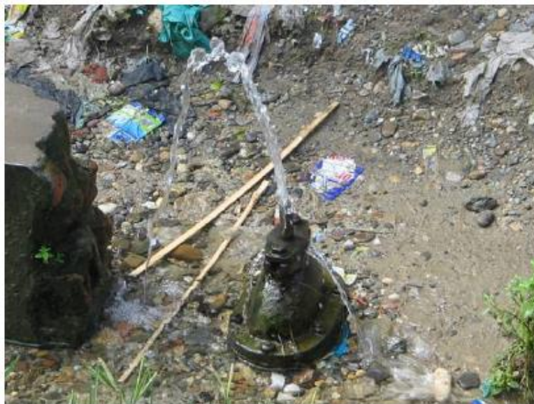
Fig. 6.1 : Water loss from supply line
