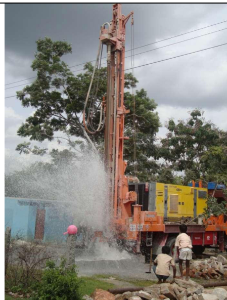
Fig. 9a: High drilling discharge at deeper fracture encountered at Sasalu EW site
