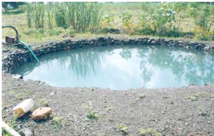
Figure 2. A recharged open well with pump for irrigation at Shekta watershed, Maharashtra.
