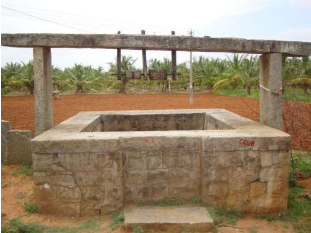
The typical dug well at B.Hosahalli village
