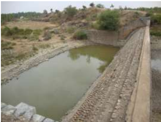
Major check dam at Ankasandra village
