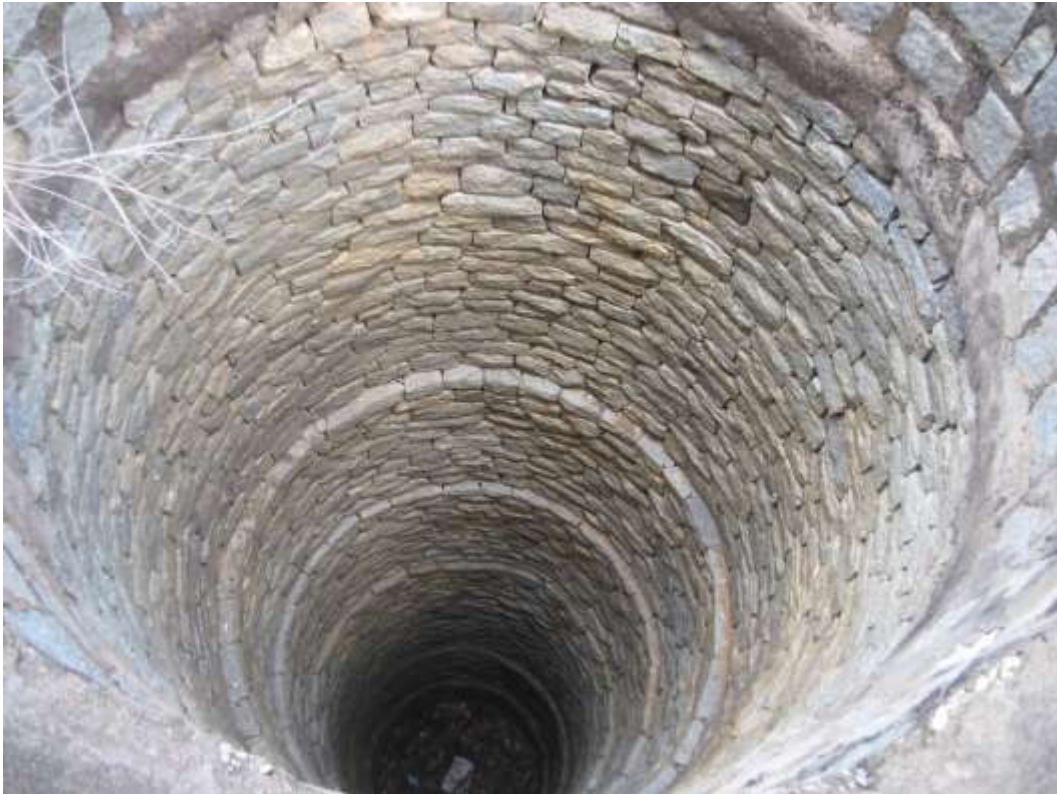
Dry dug well at Siddaramanagara village
