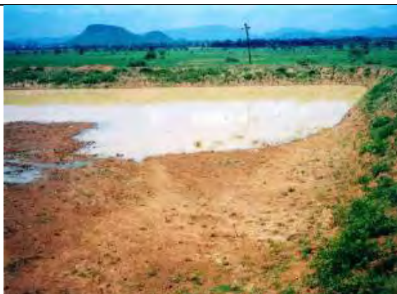
A. Barkatia Water Shed – Percolation Tank
