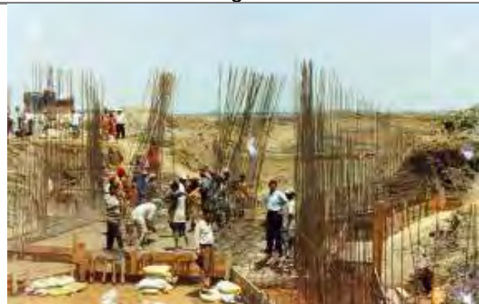
E. Kuhali-Baupokhari Sluice – Reinforcement Details
