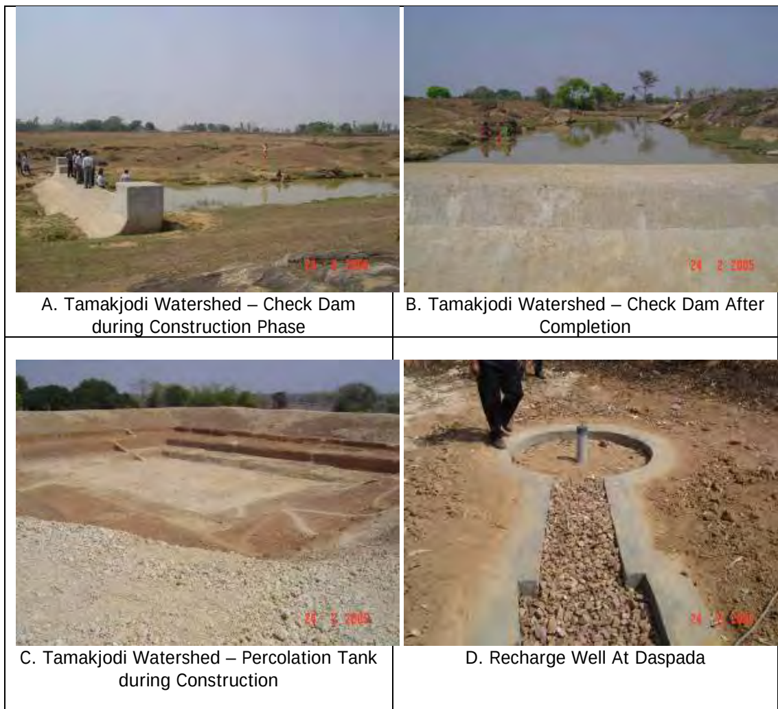
Figure 56 (A-D) : Artificial recharge structures, Tamkajodi Watershed, Saharpada Block, Keonjhar District
