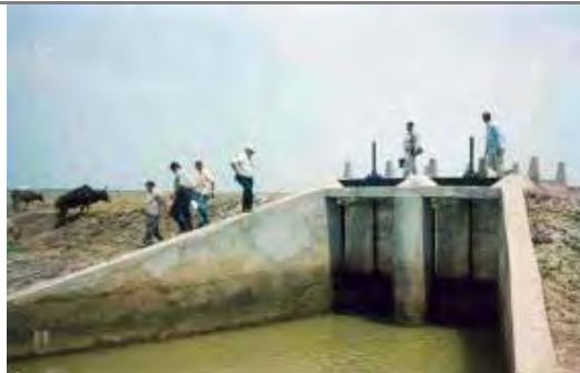
H. View of Karanjadia Sluice after Completion
