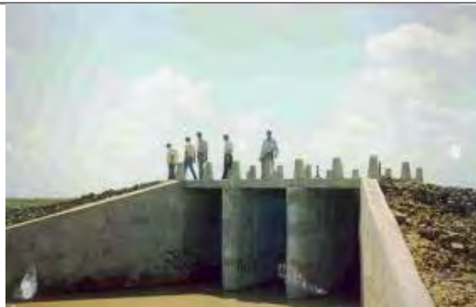
F. View of Andola Sluice after Completion
