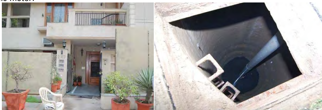
Figure.23. RTRWH & AR structure constructed at Defence colony, New Delhi
