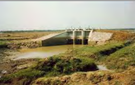
G. View of Gahamnali Sluice after Completion
