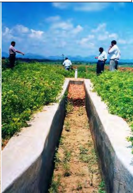
D. Barkatia Watershed - Trench with recharge Bore
