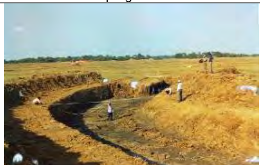
C. Sashikadeipur Creek – Excavation in Progress
