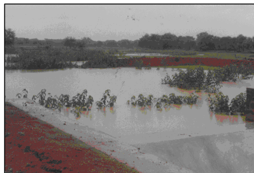
Figure. 6 Percolation tank at Tarri
