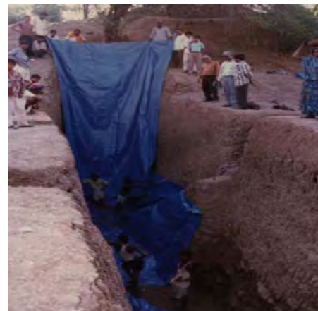
Figure.28. Subsurface Dykes at Londri Nala, District Dewas
