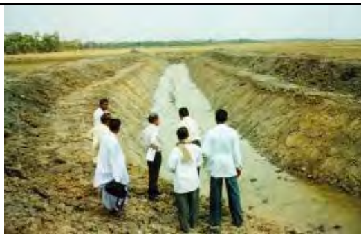
B. Ricket Chattara Creek – After Completion of Excavation
