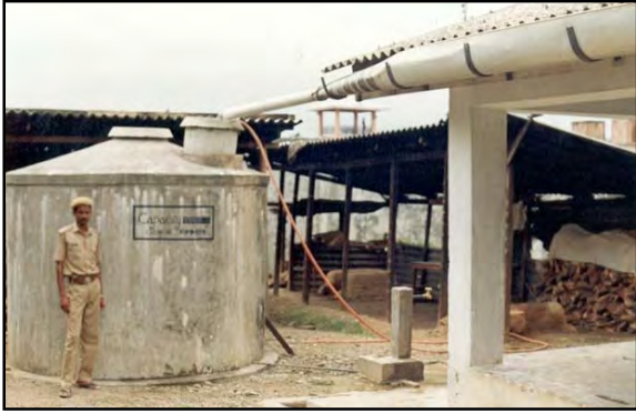
Fig-78 Rainwater harvesting tank in Portblair Jail
