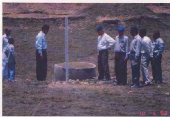
Figure.30 Recharge Shaft at Mendkikhak District Dewas
