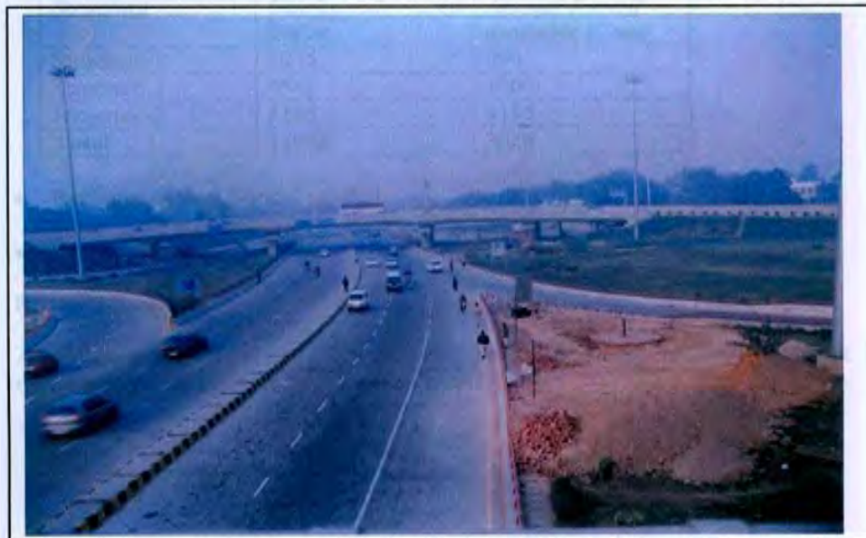
Figure.15 Artificial Recharge Structure at AIIMS Fly-over
