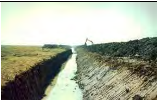
A. Ricket Chattara Creek – Excavation in progress
