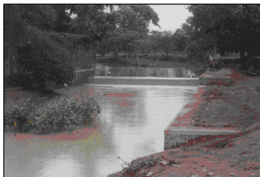
Figure.5 Check dam at Mehra kala
