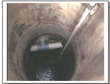
Abandoned Dug Well fitted with Rain Water Harvesting Mechanism
