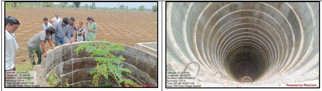
Fig. 9.3 Dug wells with depth upto 30m running dry in Pota village near mining area.
