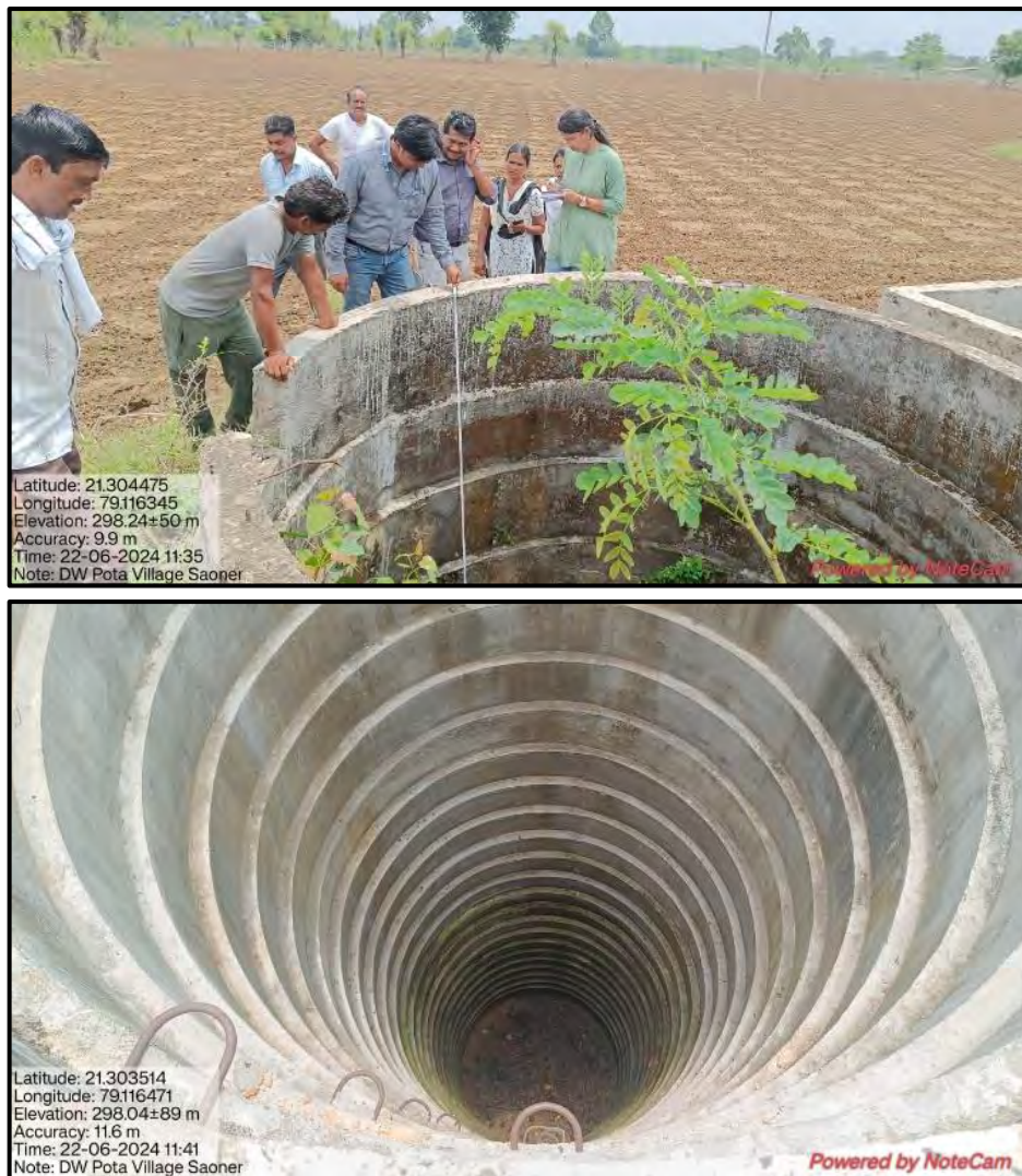
Fig.8.3 (a-b): - Field photograph of Dry dug wells (depth 30 m), Pota village, Saoner Block.
