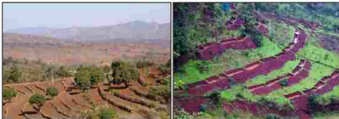
Figure-12.4: Contour/Staggered Contour trenches
