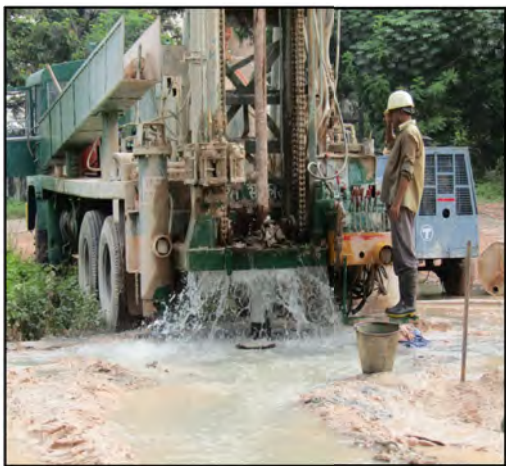
Fig 4.5: Exploratory well at Trikkakara, Kerala yielding 50400 lph
