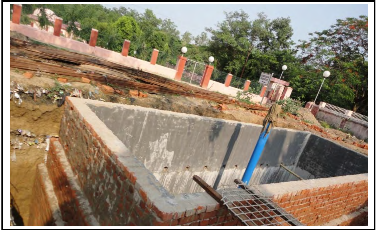
Fig. 11.1: Construction of Recharge Pit near New Petroleum Engg. Building, ISM campus Dhanbad (Side View)
