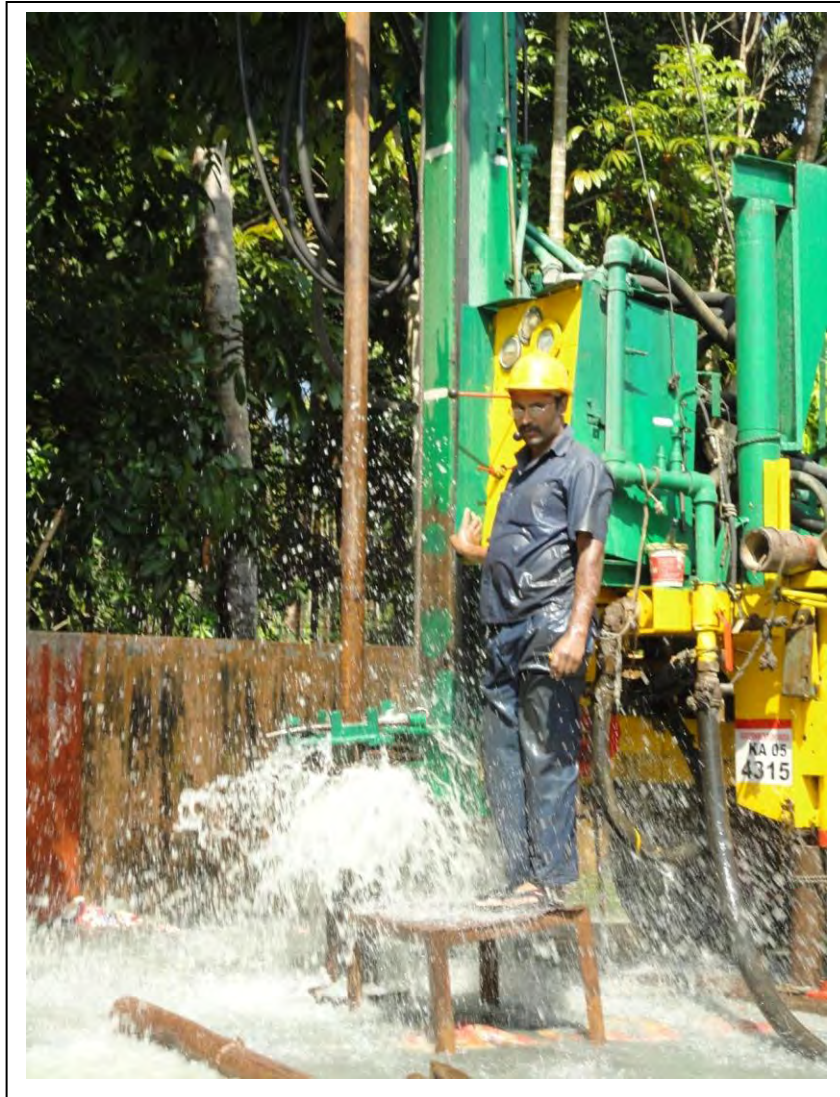
High Discharge Exploratory well at Vellikulangara, Thrissur
