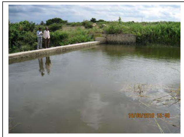
Check Dam constructed in Malur taluk under Demonstrative Projects at SWR, Bangalre
