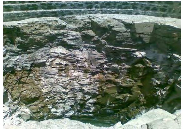
Dug well showing fractured aquifer system in RHS area of Jalna District
