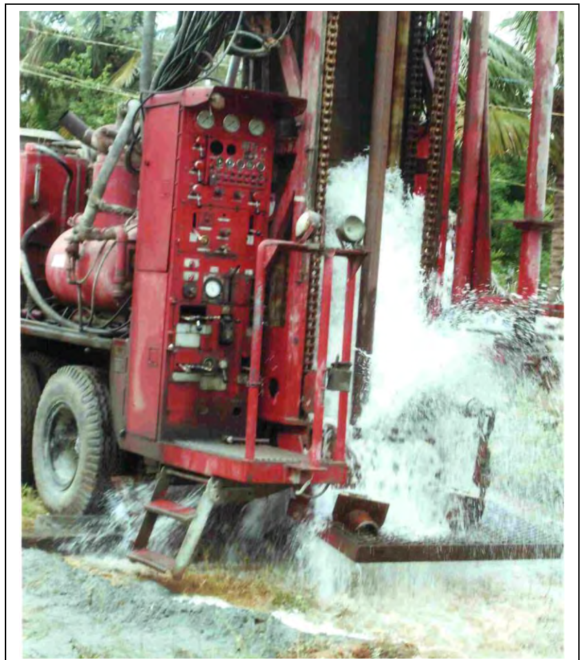
Free flow exploratory tube well drilled at Karaikurichy in the Neyveli Hydrogeological Basin, Ariyalur district tapping Cuddalore sandstone
