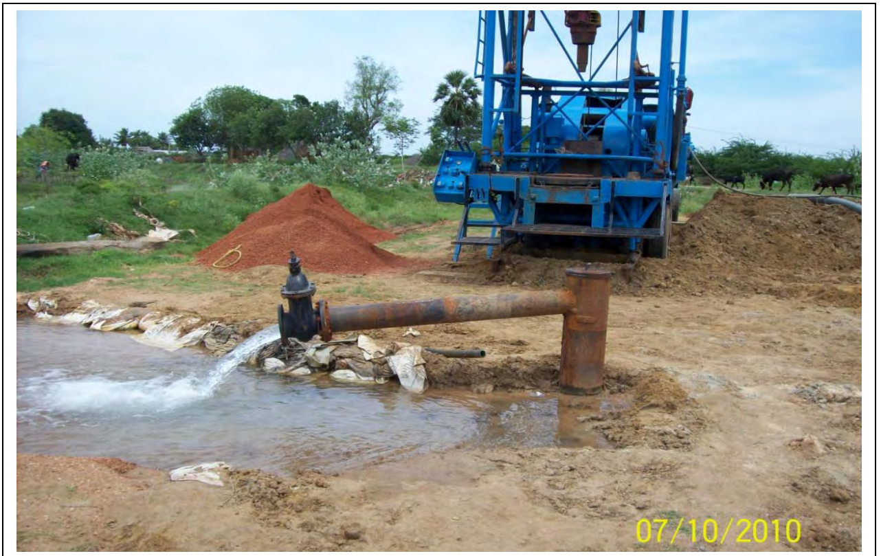
Free flow exploratory tube well drilled at Karaikurichy in the Neyveli Hydrogeological Basin, Ariyalur district tapping Cuddalore sandstone
