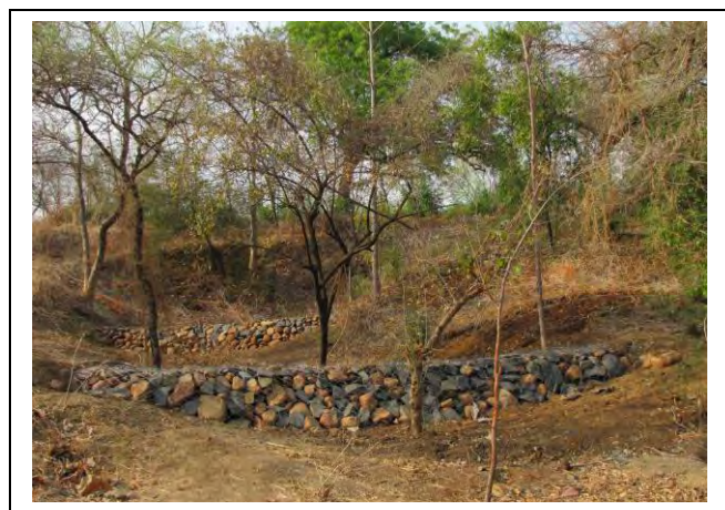
Artificial Recharge and Rainwater harvesting Studies under CSS (XI th Plan) at Rajbhavan at Nagpur
