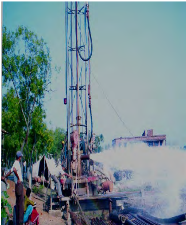
Deep exploratory Well constructed by CGWB, at Khasbalanda village, Haroa block, North 24 parganas district, West Bengal using cement sealing techniques
