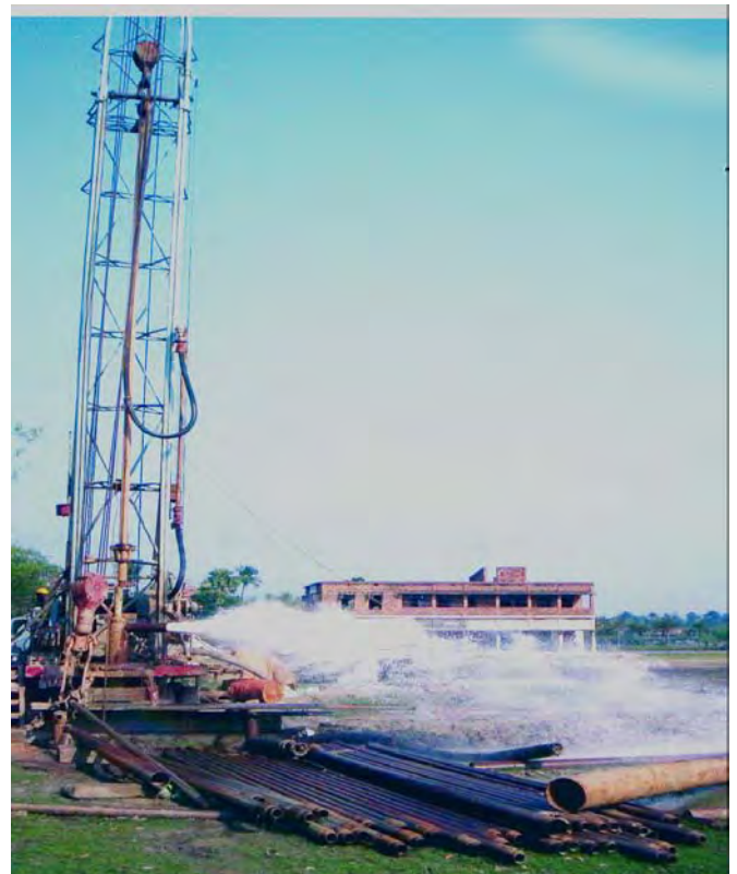
Deep exploratory Well constructed by CGWB, at Khasbalanda village, Haroa block, North 24 parganas district, West Bengal using cement sealing techniques ( cement sealing depth 100 to 105 m bgl ) tapping the deeper arsenic free aquifer (175 to 205 m bgl) yielding 34 lps of arsenic free water.
