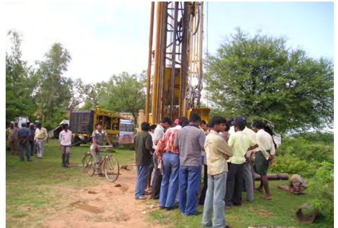
Trainees at Drilling Site
