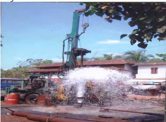
One high yielding PZ constructed at Pangh, Malappuram district with discharge 10 lps, depth 184.50 mtrs and geology: Khondalite.
