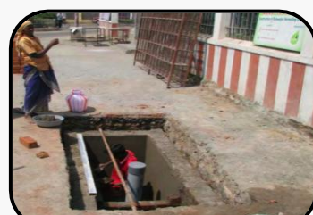
Trench with Borewell
