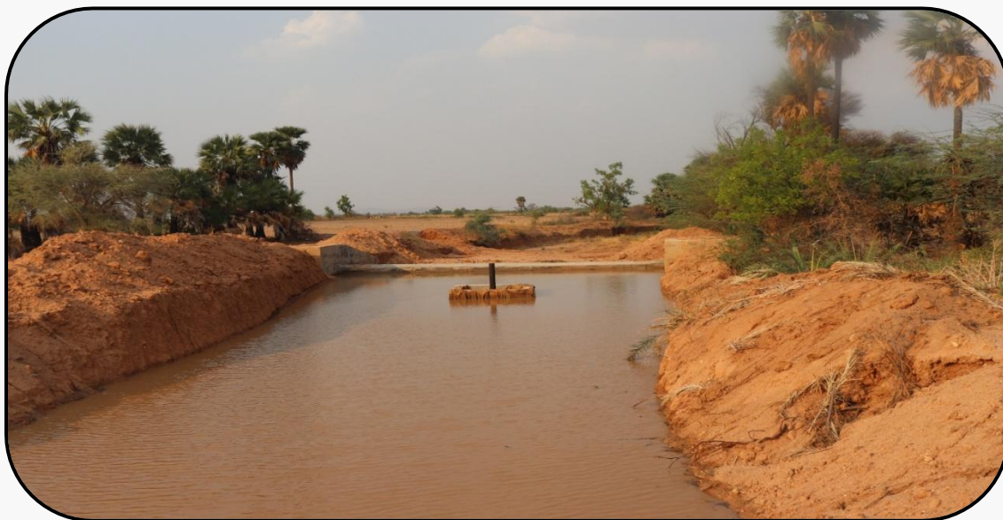
Percolation tank with Recharge shaft
