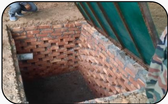
Sub-Surface Technique: Recharge Pit
