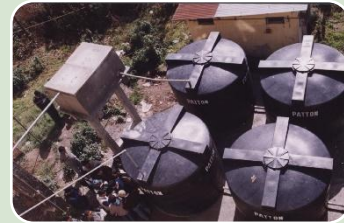
Harvesting of roof water in tanks
