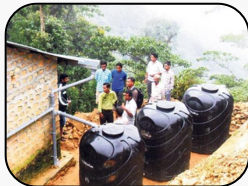
Roof Top Rainwater Harvesting
