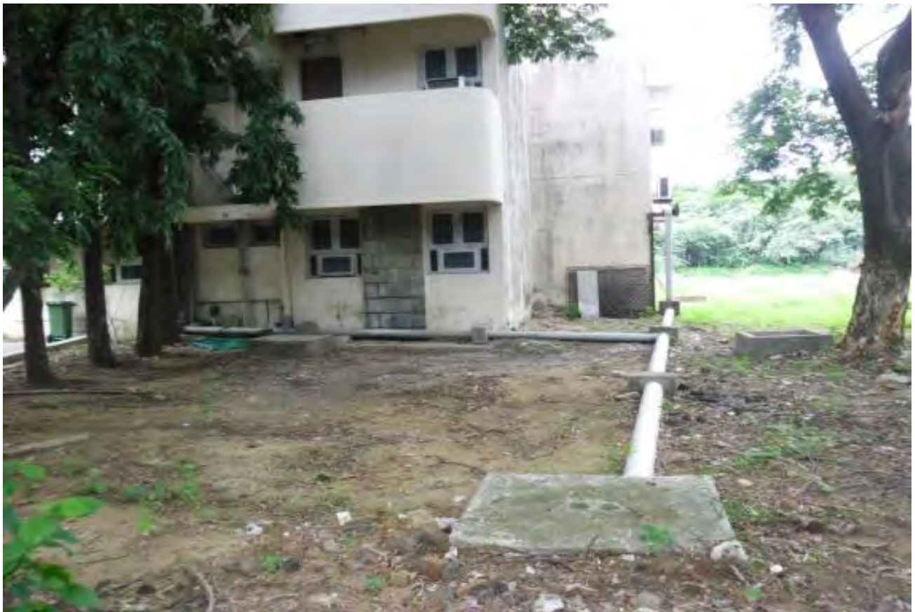
Collection, conveyance and Filtering Unit of roof top rainwater harvesting Rain water Harvesting in the premises of the NITTTR, Taramani, Chennai city, Tamil Nadu.
