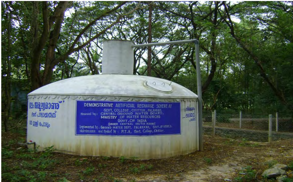
A view of the functional Ferro Cement TankFerro Cement Tank with Recharge Pit
