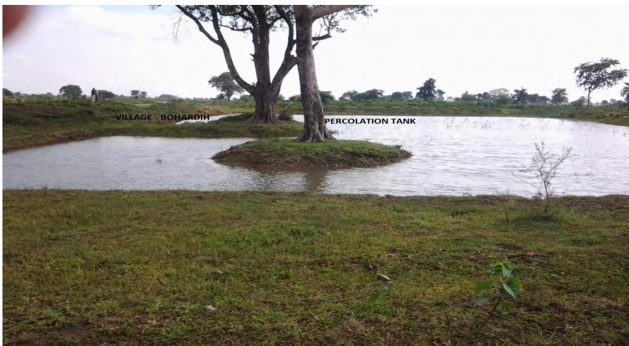
Percolation tank at Bohardih
