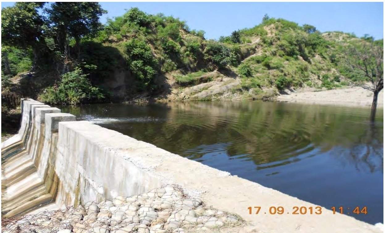
CHECK DAM AT PHANGERI, KATHUA
