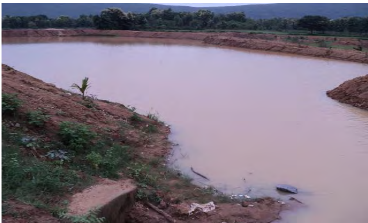
Post-Project Recharge Tank, Burudi Watershed, Ganjamblock, Odisha
