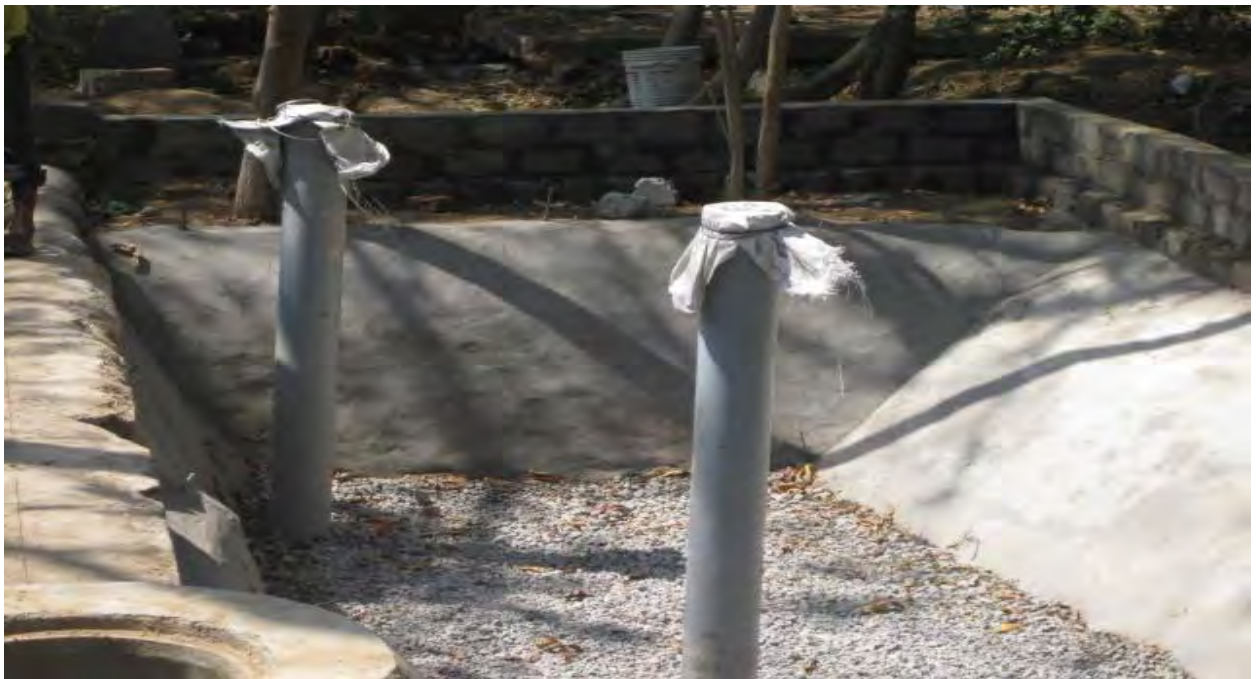
Open pond along with two recharge wells at Jawaharlal Nehru Technological University(JNTU), Kukatpaali Hyderabad, Ranga Reddy dist, Telangana
