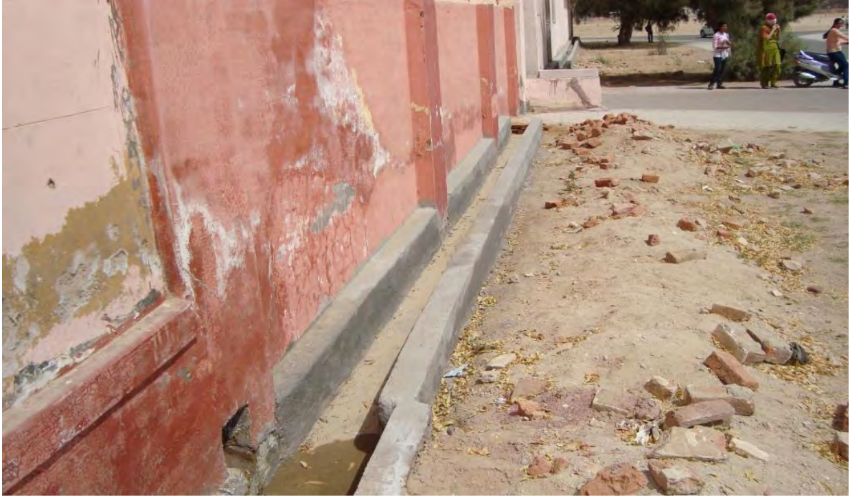
Channel for roof top run off collection Govt. Polytechnical Collage (Boys), Bikaner city, Dist Bikaner
