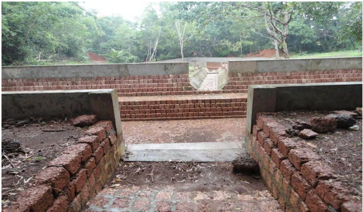
A view of Channels connecting silt tank to Recharge Pit Roof Top Rain Water Harvesting at Kendriya Vidyalaya No. 2, Vidyanagar, Kasargoddist, Kerala
