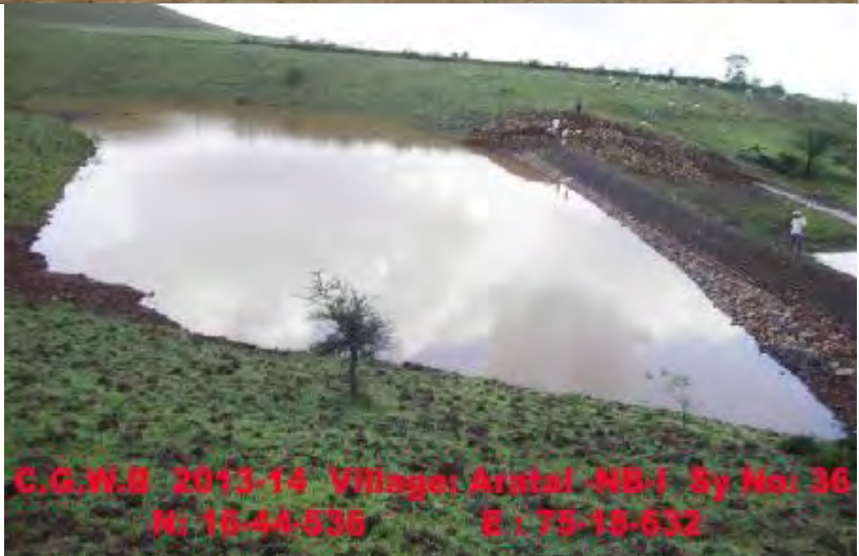
Nala bund constructed in the sub watershed, Arthal Water Shed Artificial Recharge in Arthal Water Shed, Athni Block Belgavi District, Karnataka
