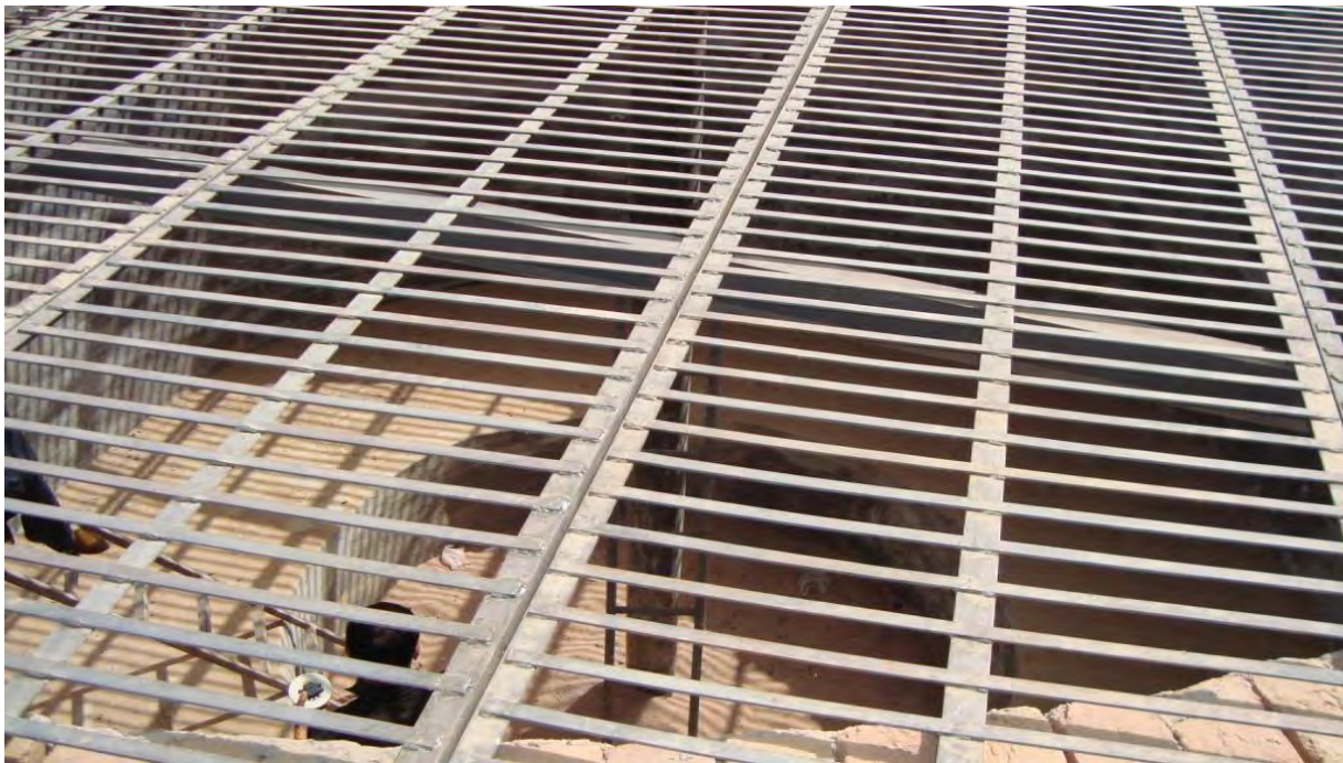
Circular Recharge Pit with filter pit & recharge tube well Govt. MahilaPolytechnical Collage, Bikaner city, Dist Bikaner
