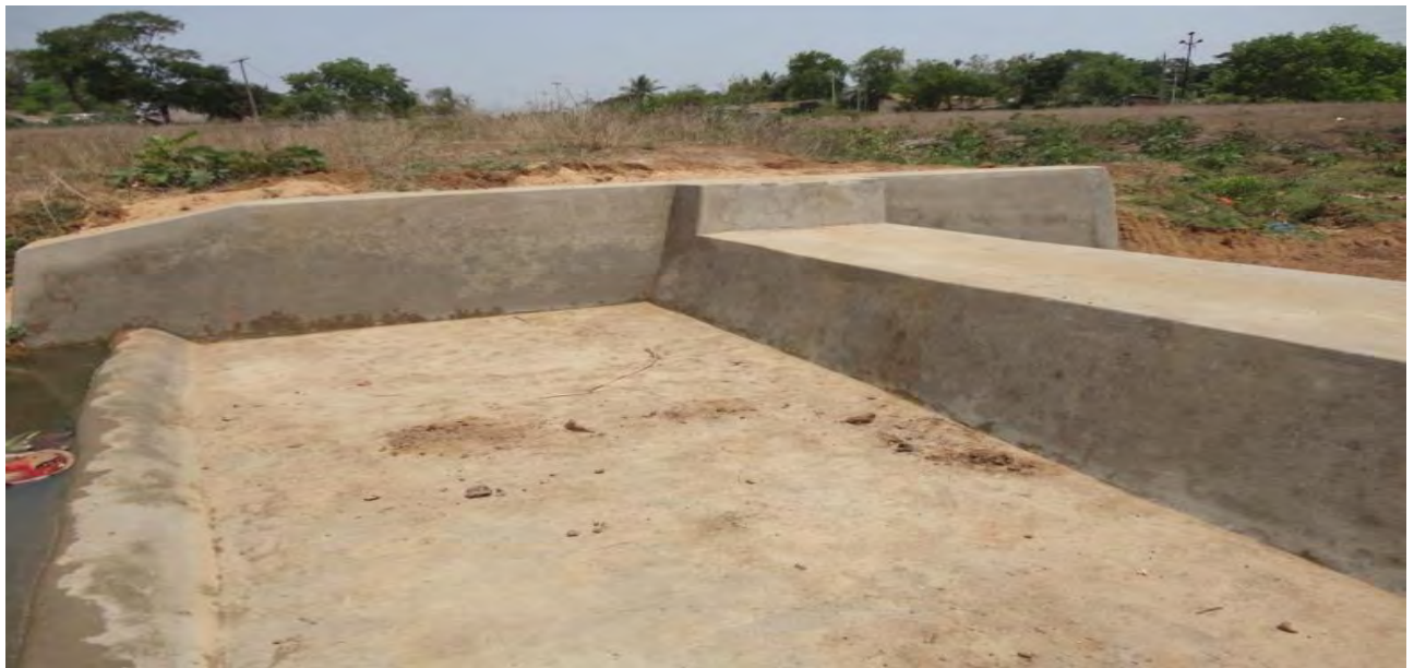
CHECK DAM OVER GANDA NALLAH
