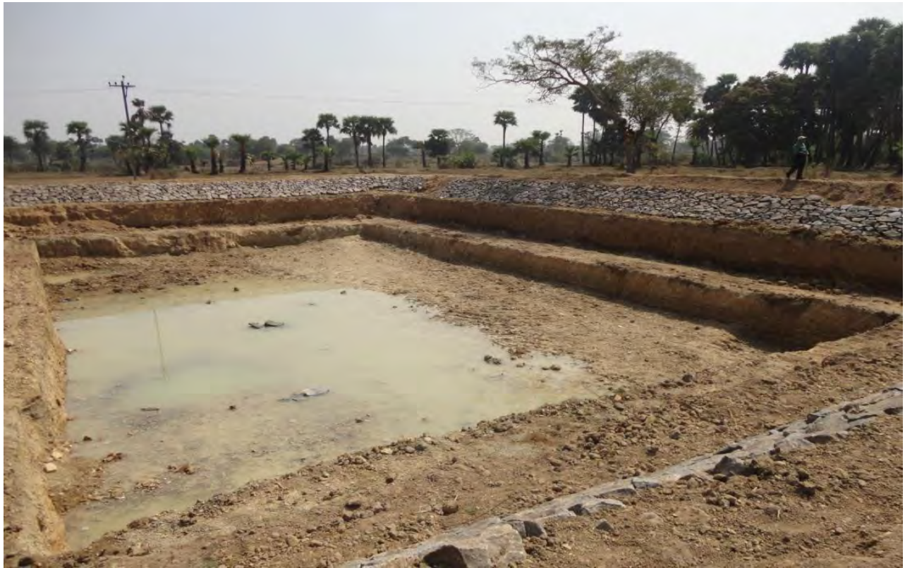
RECHARGE TANK AT NUASAH-I -Ligarkat Watershed, Banerpal block, AngulDist, Odisha
