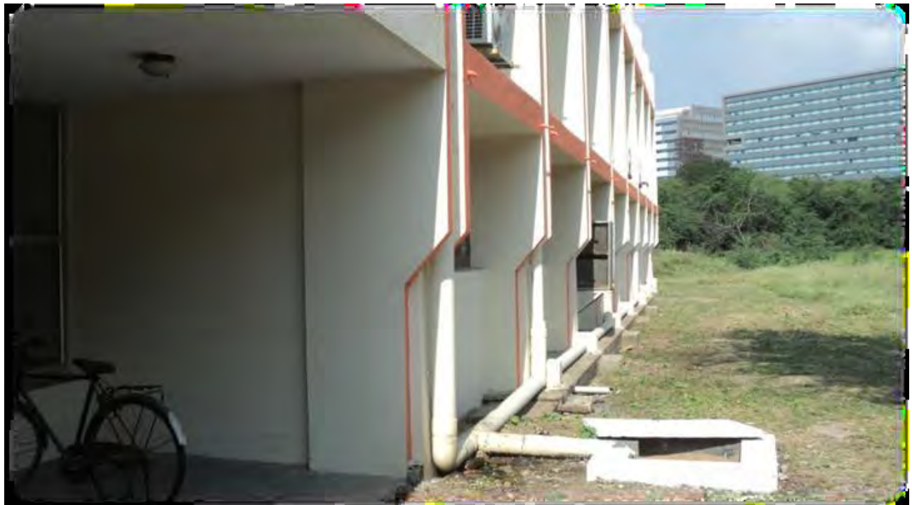
Collection, conveyance and Filtering Unit of roof top rainwater harvesting Rain water Harvesting in the premises of the NITTTR, Taramani, Chennai city, Tamil Nadu.
