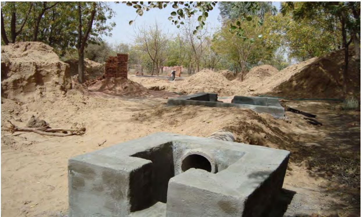
De-silting Pit- Govt. Polytechnical Collage (Boys), Bikaner city, Dist Bikaner
