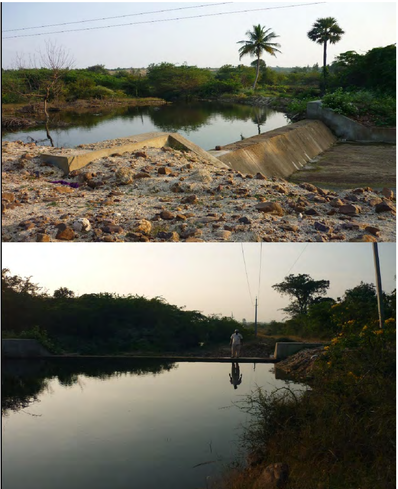
Check Dam at Mittoor Village Artificial Recharge Structures on ground water in Chittoor District, Andhra Pradesh
