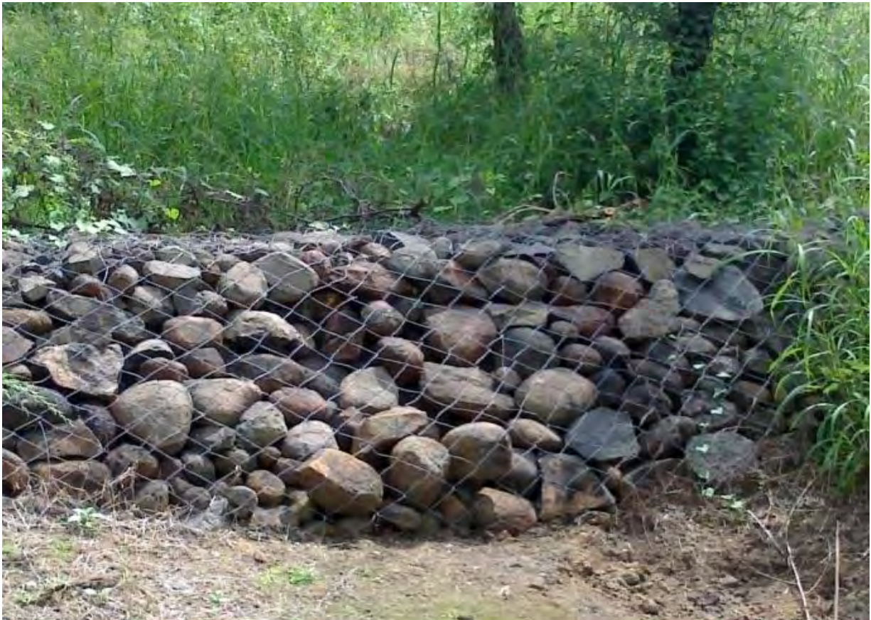
Gabion Structure-After monsoon Artificial Recharge to Groundwater in Raj Bhawan area, Nagpur, Maharashtra
