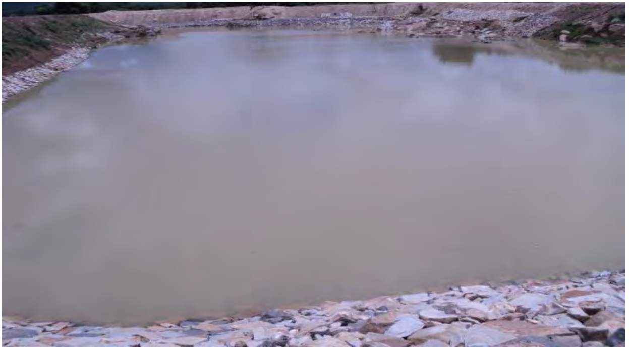
Post-Project Recharge Tank, Burudi Watershed, Ganjamblock, Odisha
