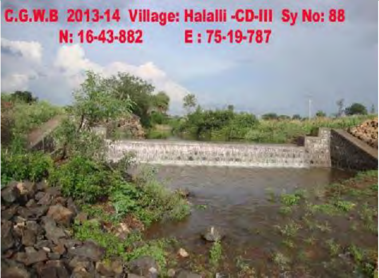
Check dams constructed in the sub watershed, Arthal Water Shed Artificial Recharge in Arthal Water Shed, Athni Block Belgavi District, Karnataka
