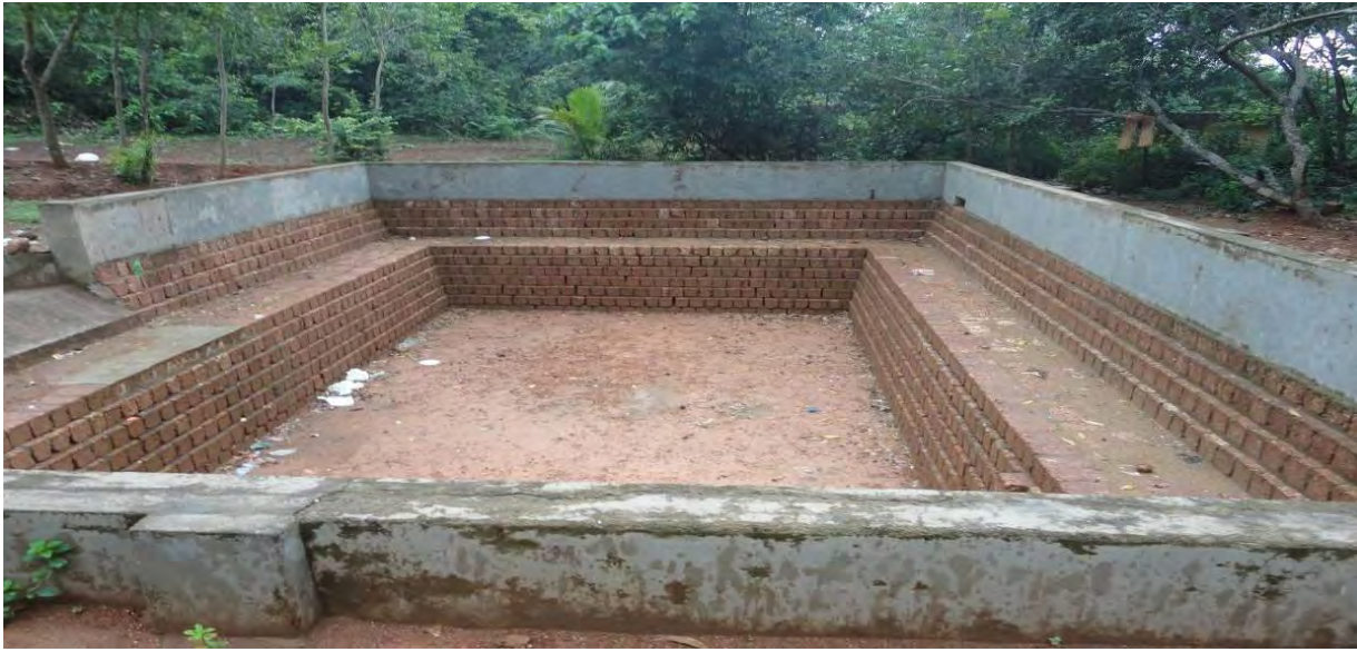
A View of Recharge Pit
