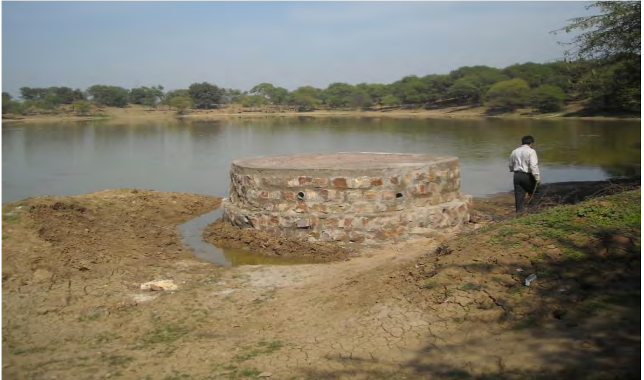
Recharge Shaft no. 1 at village Kanwar
