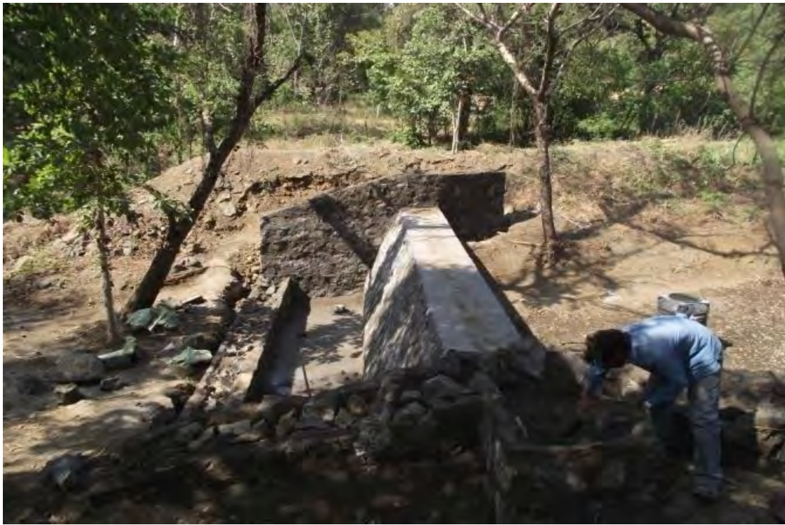
Cement Nala Bandh-Before monsoon
