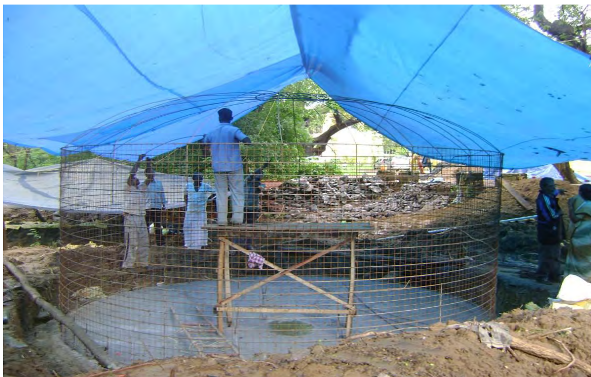
Ferro Cement Tank under construction Roof Top Rain Water Harvesting at Govt. college, Chittordist, Kerala
