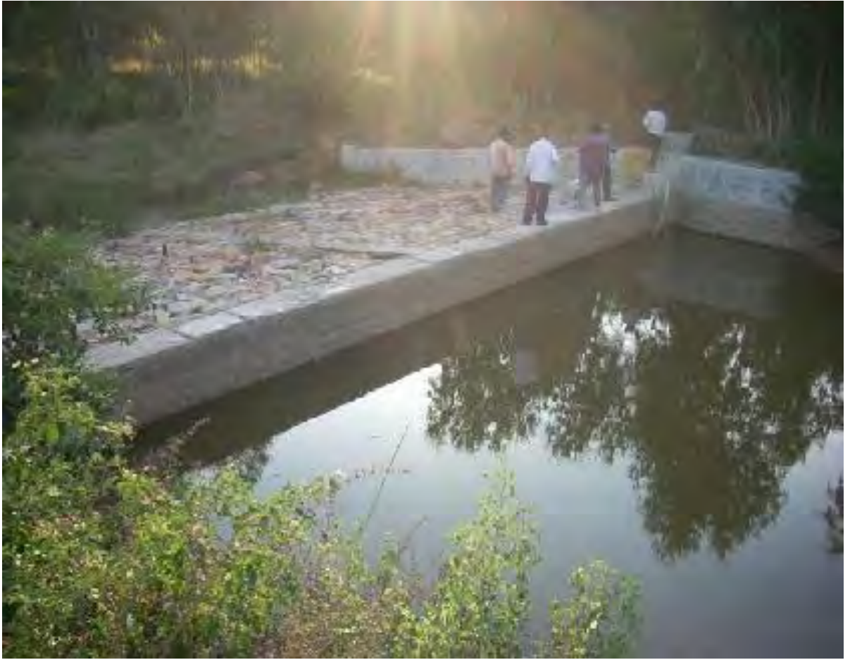
Check Dam constructed at Malur Taluk
