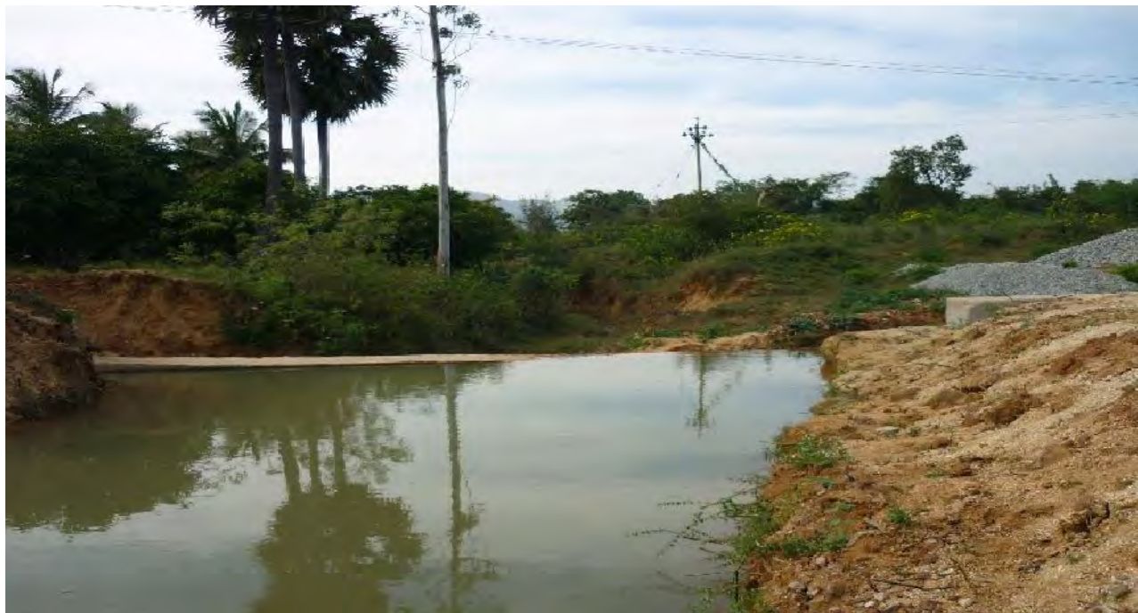
Check Dam at Karvetinagaram Village
