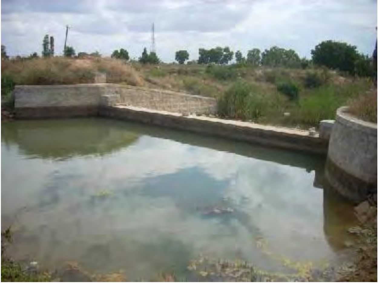
Percolation Tank constructed at Malur Taluk
