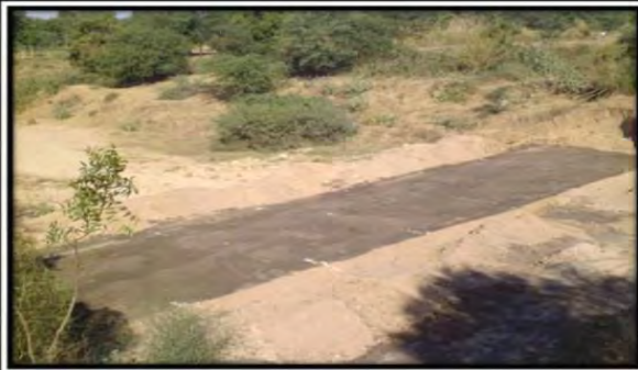
Under Ground Check Dam Village : Zanda Ta- Kapadvanj Under and After Construction
