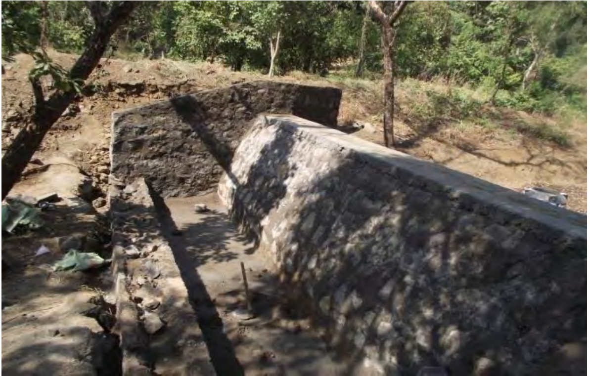
Cement Nala Bundh-Before monsoon
