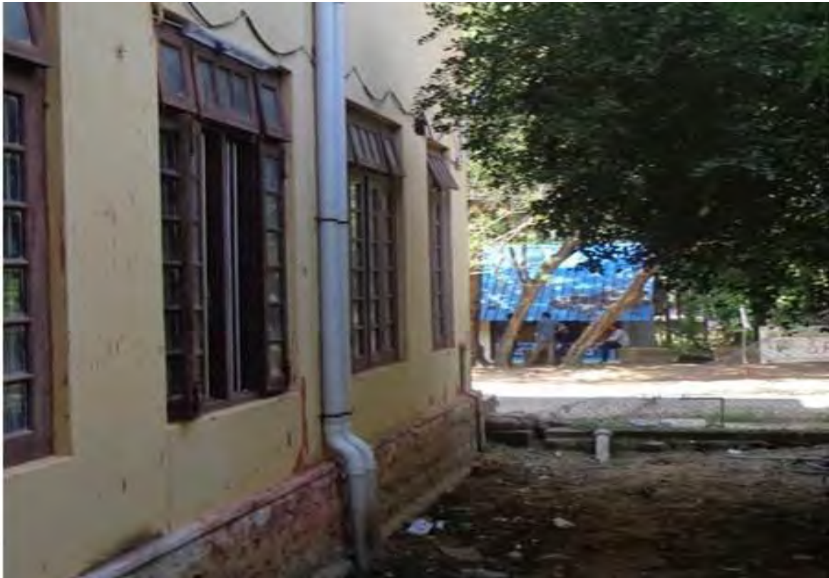
A view of the down-pipe for conveying rainwater to the storage tank. Roof Top Rain Water Harvesting at Govt. college, Chittordist, Kerala
