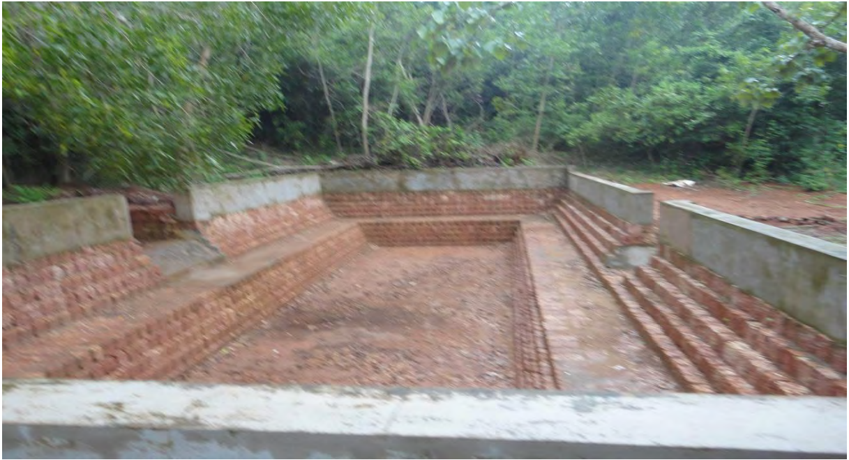
A View of Silt Collection Tank
