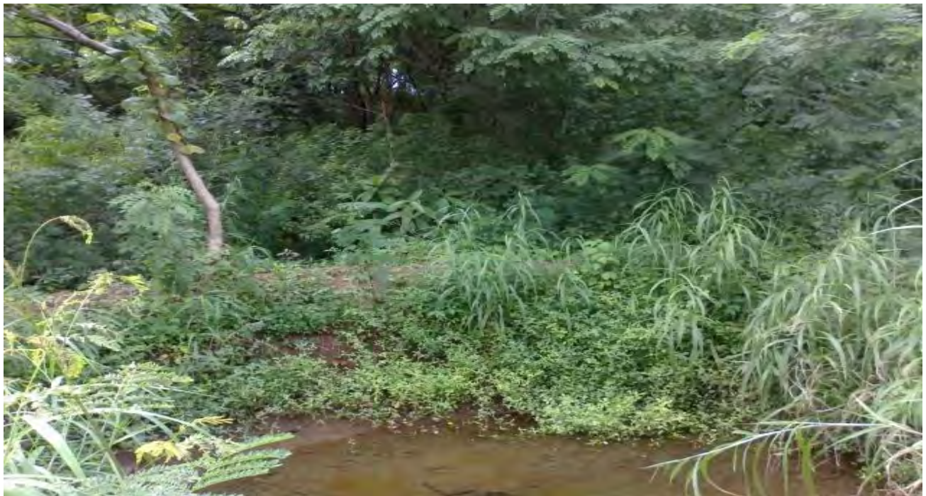
Gabion Structure-After monsoon
