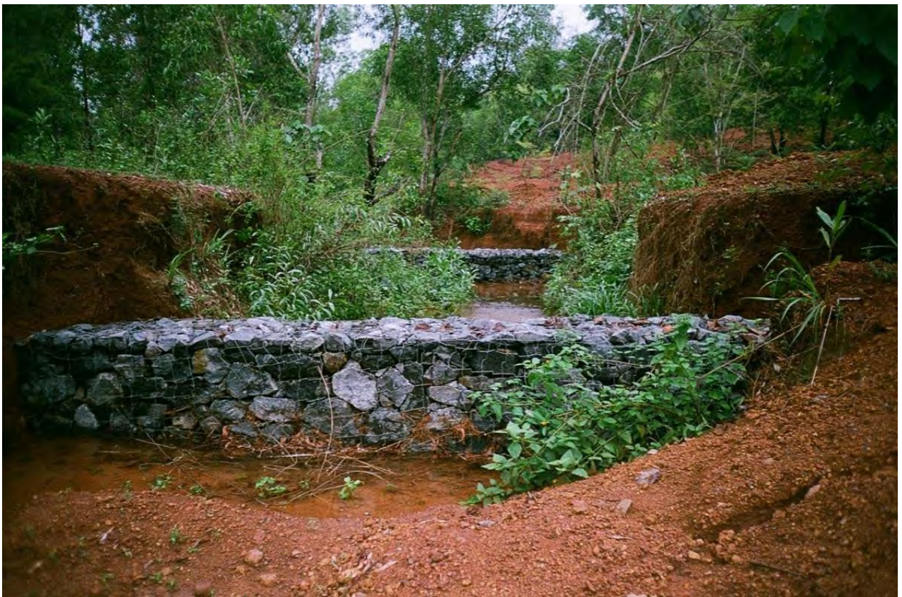
Loose Boulder Check Dam across a small stream
