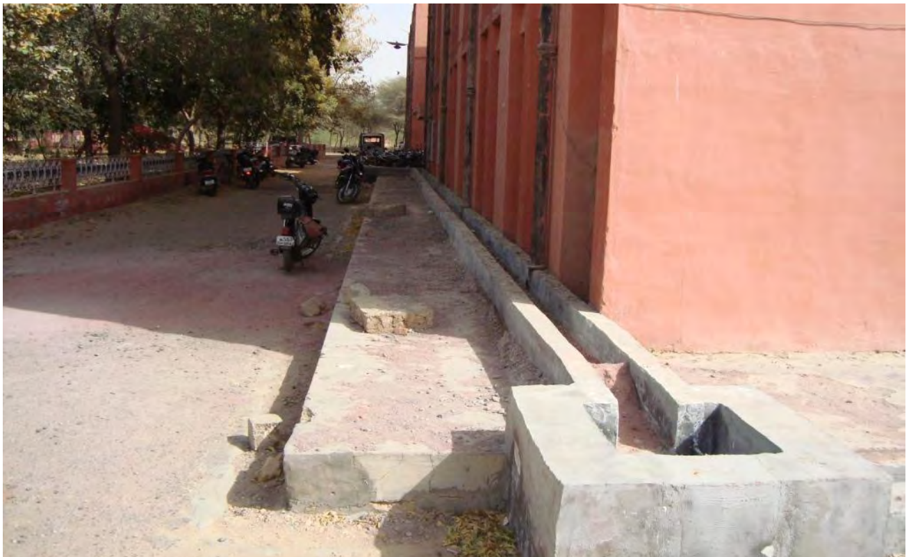
Water Channel for collection of roof top runoff-CE, IGNP Office Building, Bikaner city, Dist Bikaner
