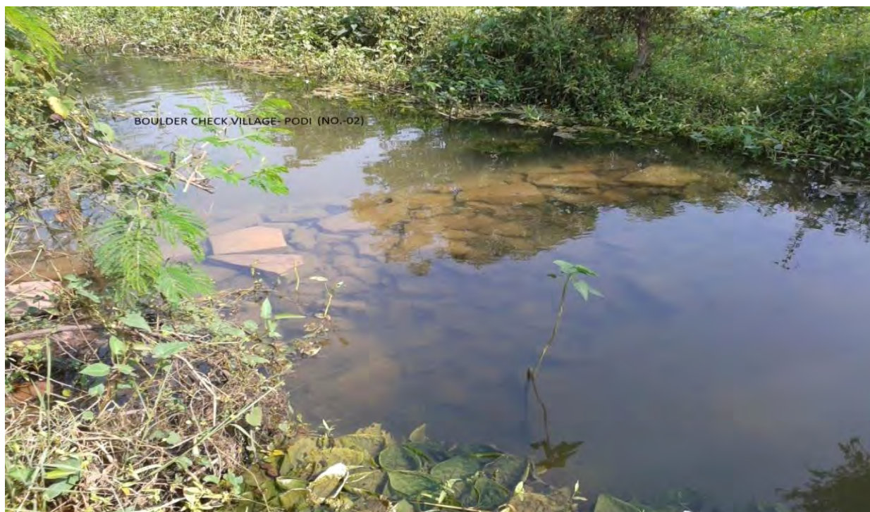
Boulder Check dam at Podi
