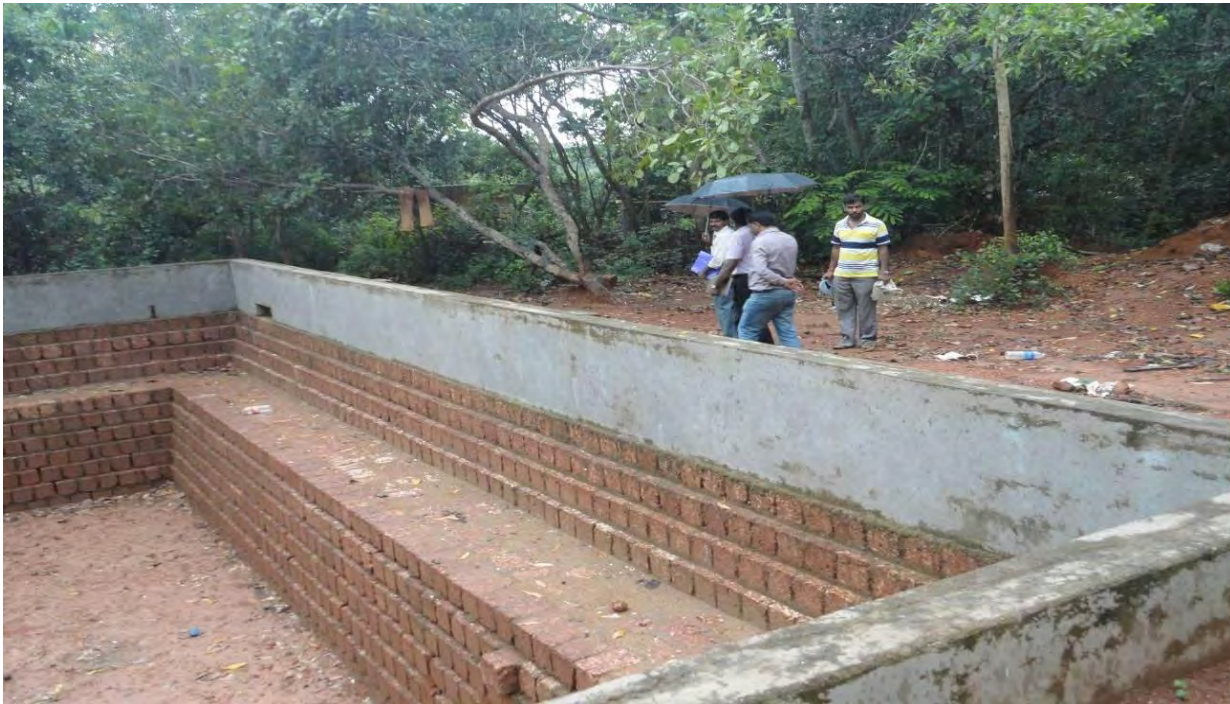
A View of Recharge Pit
