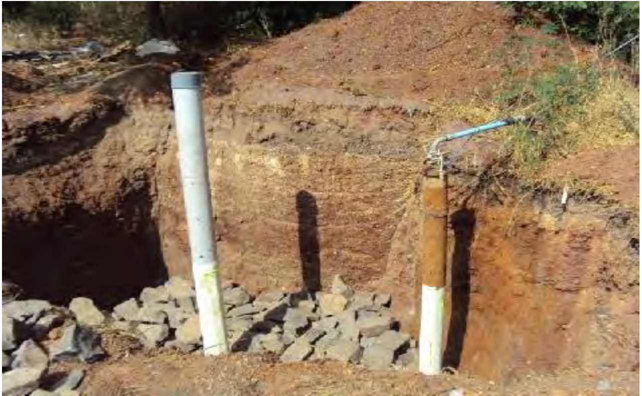
Recharge Pit Construction
