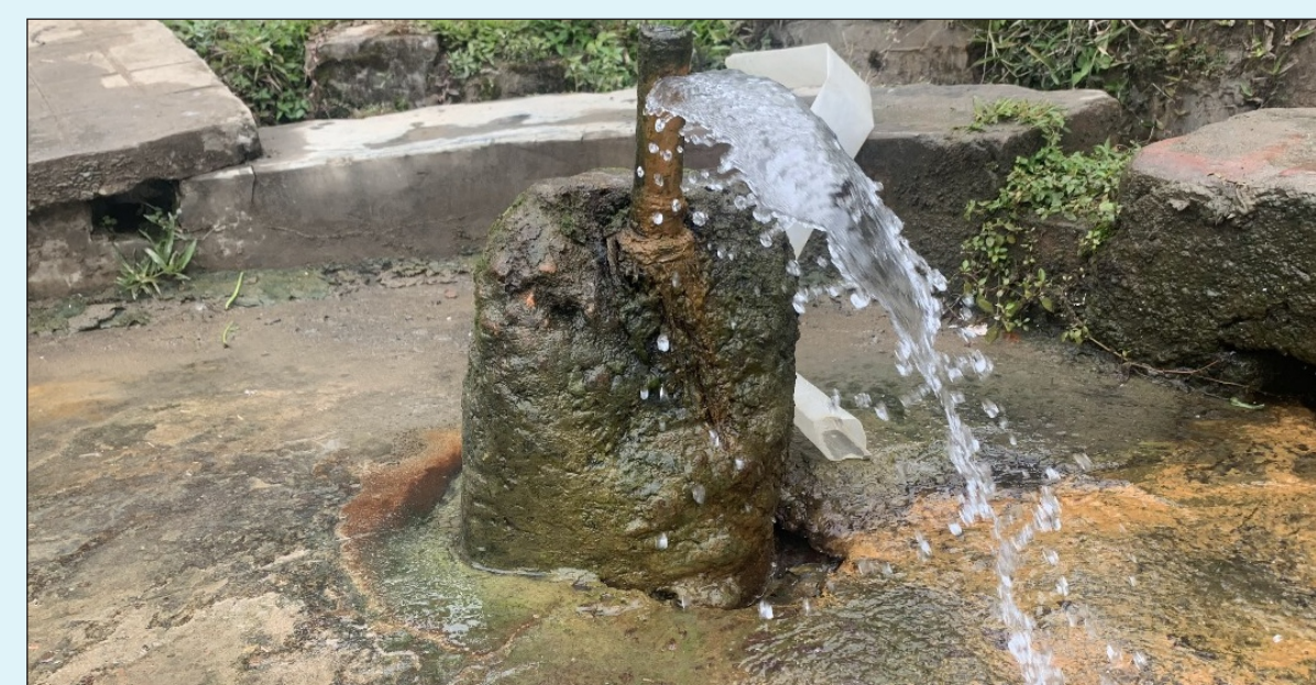
Artesian well at Khowai town, Khowai Block used for domestic purpose
