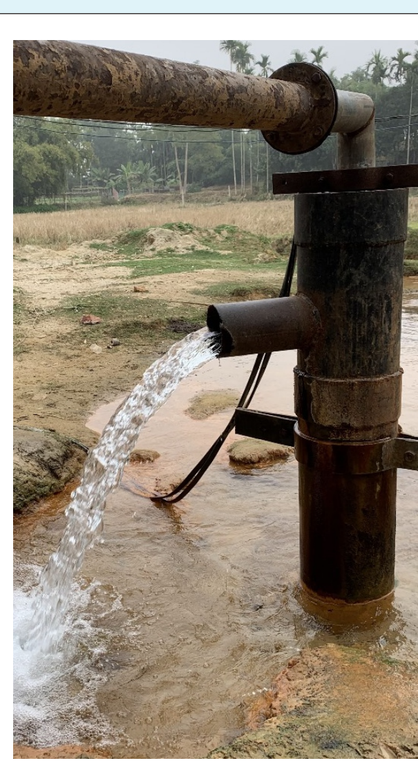
High yielding auto flow well at Char Ganki, Khowai block with a discharge of 14.6 lps
