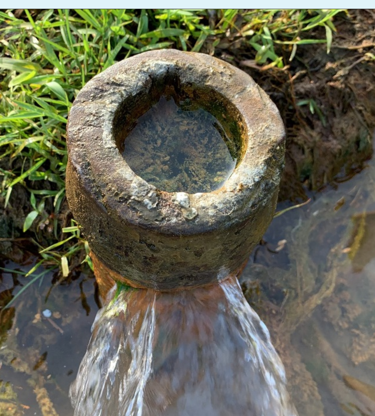
Iron deposition and slime formation at Ratia, Kalyanpur block
