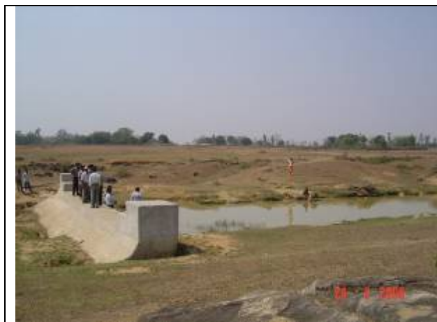
A. Tamakjodi Watershed - Check Dam during Construction Phase
