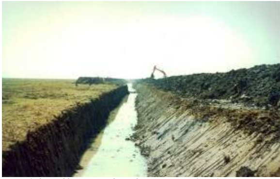
A. Ricket Chattara Creek - Excavation in progress
