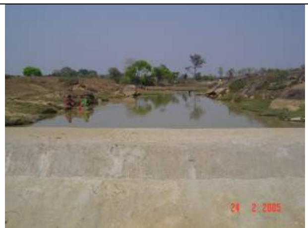
B. Tamakjodi Watershed - Check Dam After Completion
