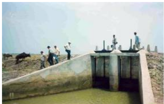
H. View of Karanjadia Sluice after Completion
