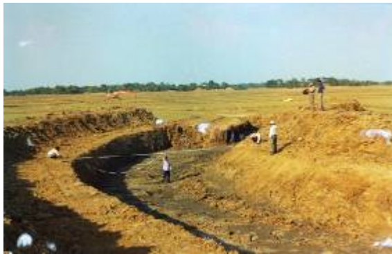
C. Sashikadeipur Creek - Excavation in Progress
