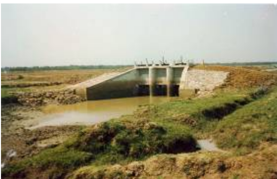
G. View of Gahamnali Sluice after Completion
