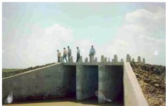
F. View of Andola Sluice after Completion
