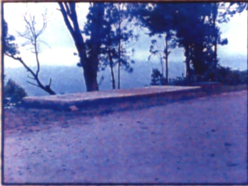
ROOF TOP RAIN WATER HARVESTING STORAGE SYSTEM
