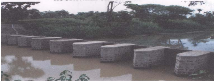
ROOPAWALI CHECK DAM
