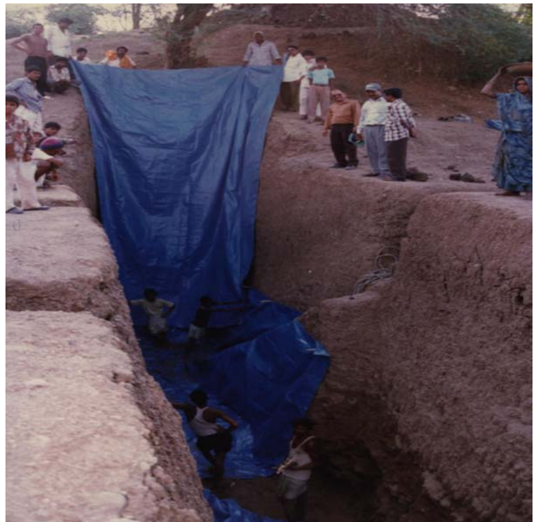
Sub Surface Dyke at Londri Nala, District Dewas.
